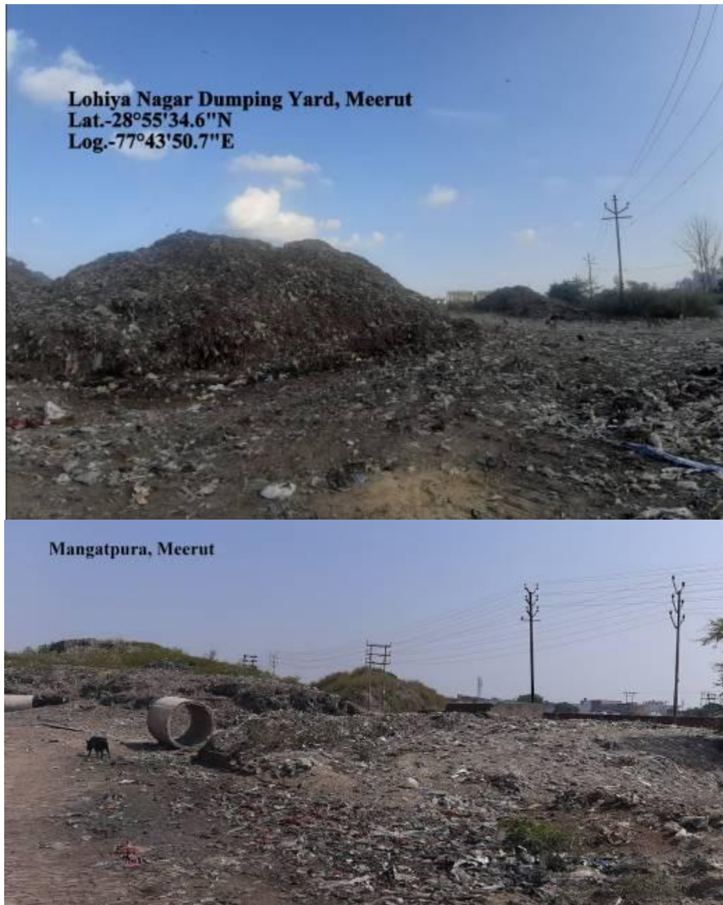
Figure 61: Solid Waste Dump Site
