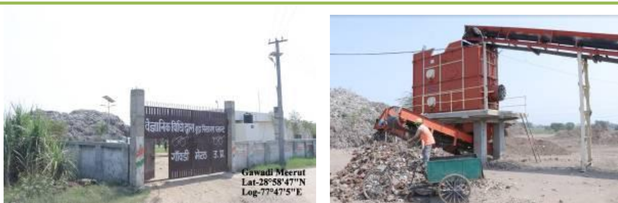
Figure 59: Solid Waste Dump Site
