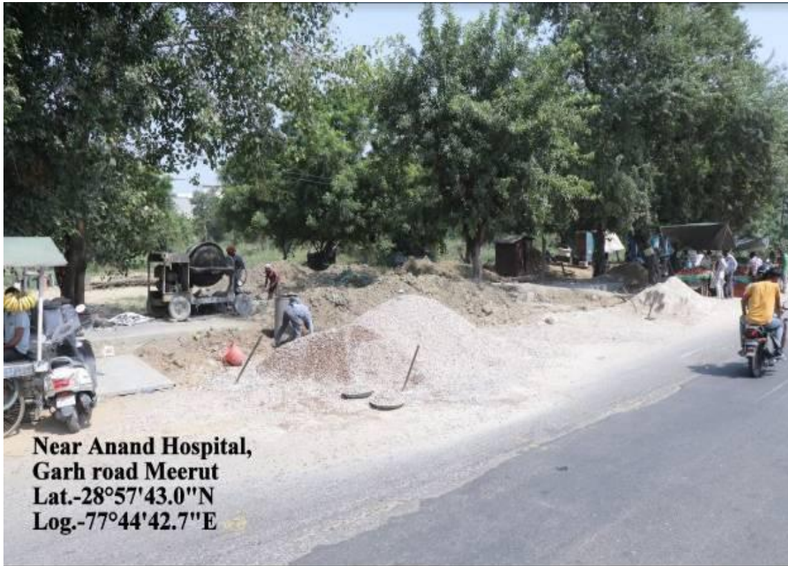
Figure 57: Construction Dust Site in Meerut City
